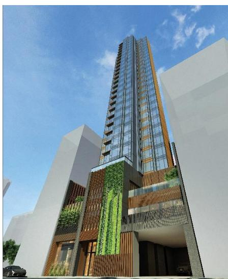
The BIM simulation of the URA's Ash Street Development Project in Tai Kok Tsui applying Concrete MiC.
